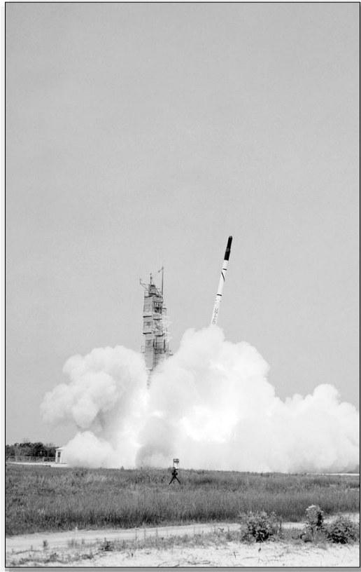
Photograph of MS-1 during one of the 43 seconds before the rocket tore itself apart.
